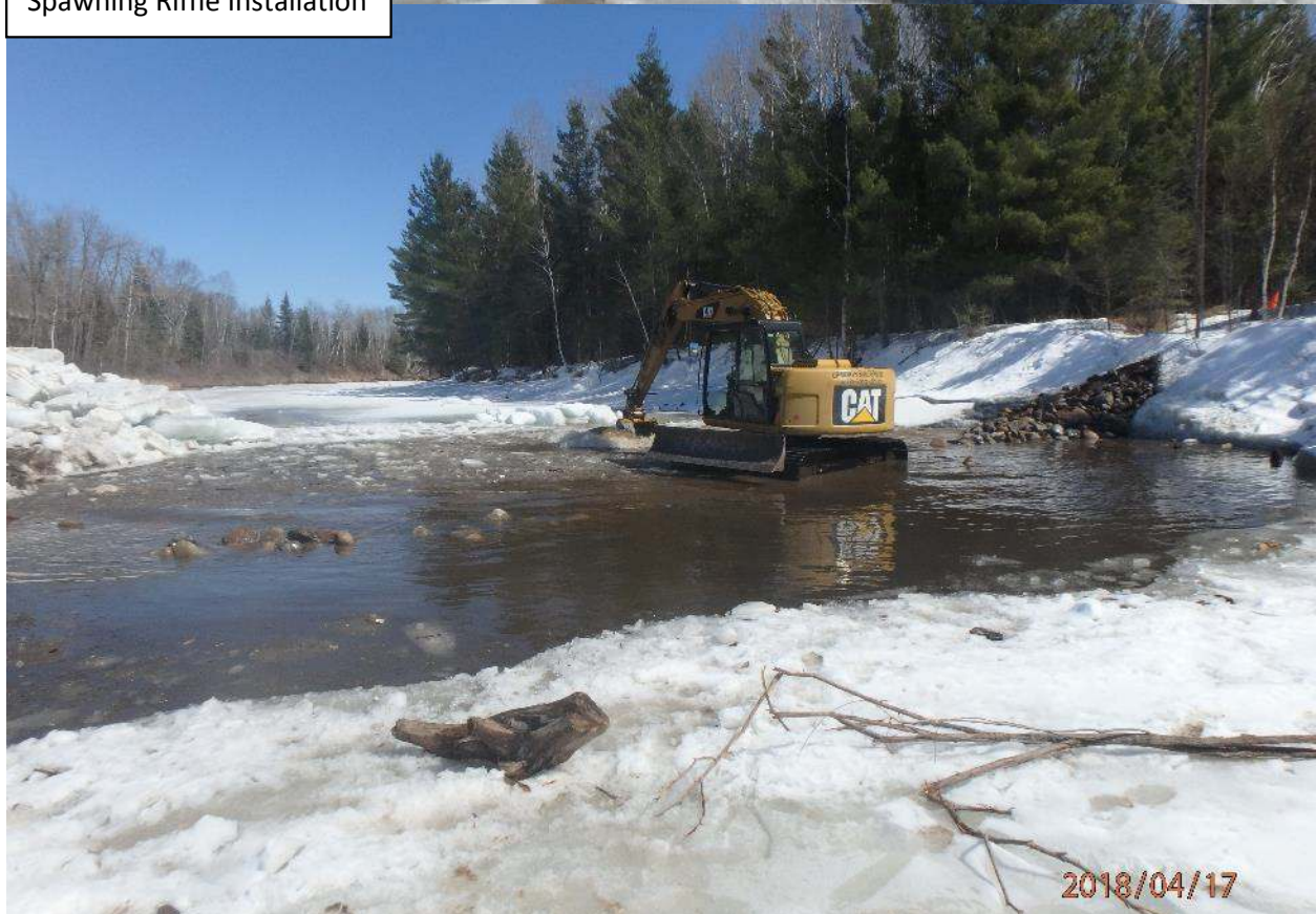
Spawning Riffle Installation
