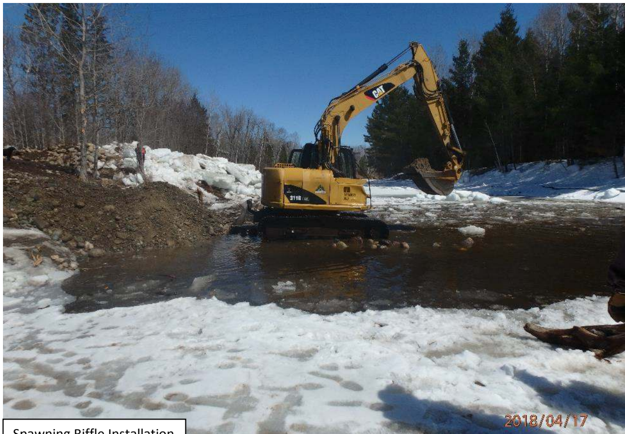
Spawning Riffle Installation
