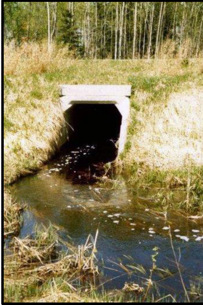
Culvert for Meadow Brook flowing from the west to east side of property under Highway 71
