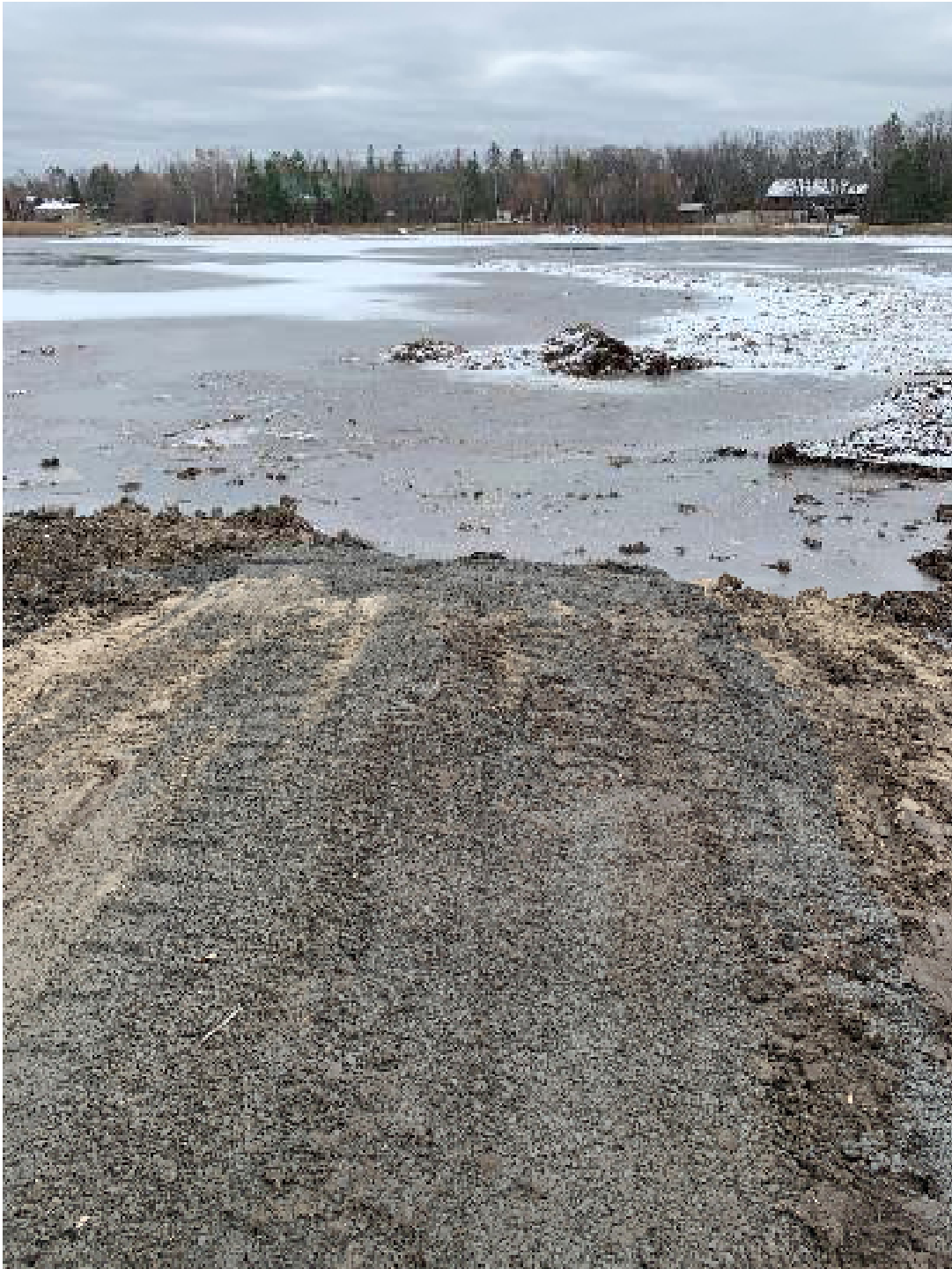
Figure 25 Resurfaced public access. Photo taken 11/2/2023
