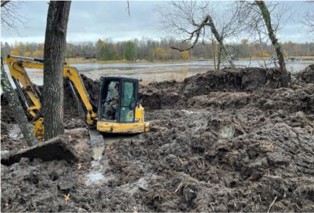
Figure 19 Biomass piled at the public access. Photo taken on 10/24/2023.
