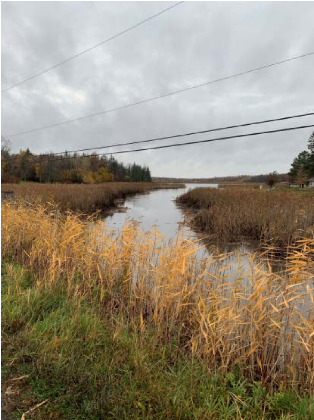
Figure 16 Temporary solution - 16ft channel cut through for additional water flow to the culvert on the western portion of the restoration site.
