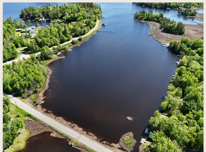
After cutting, prior to road and culvert work.
