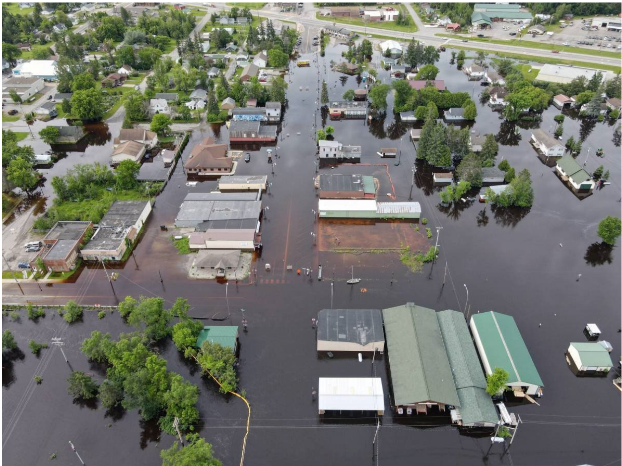
Figure 2. Flooding in Cook, MN on June 21, 2024.
