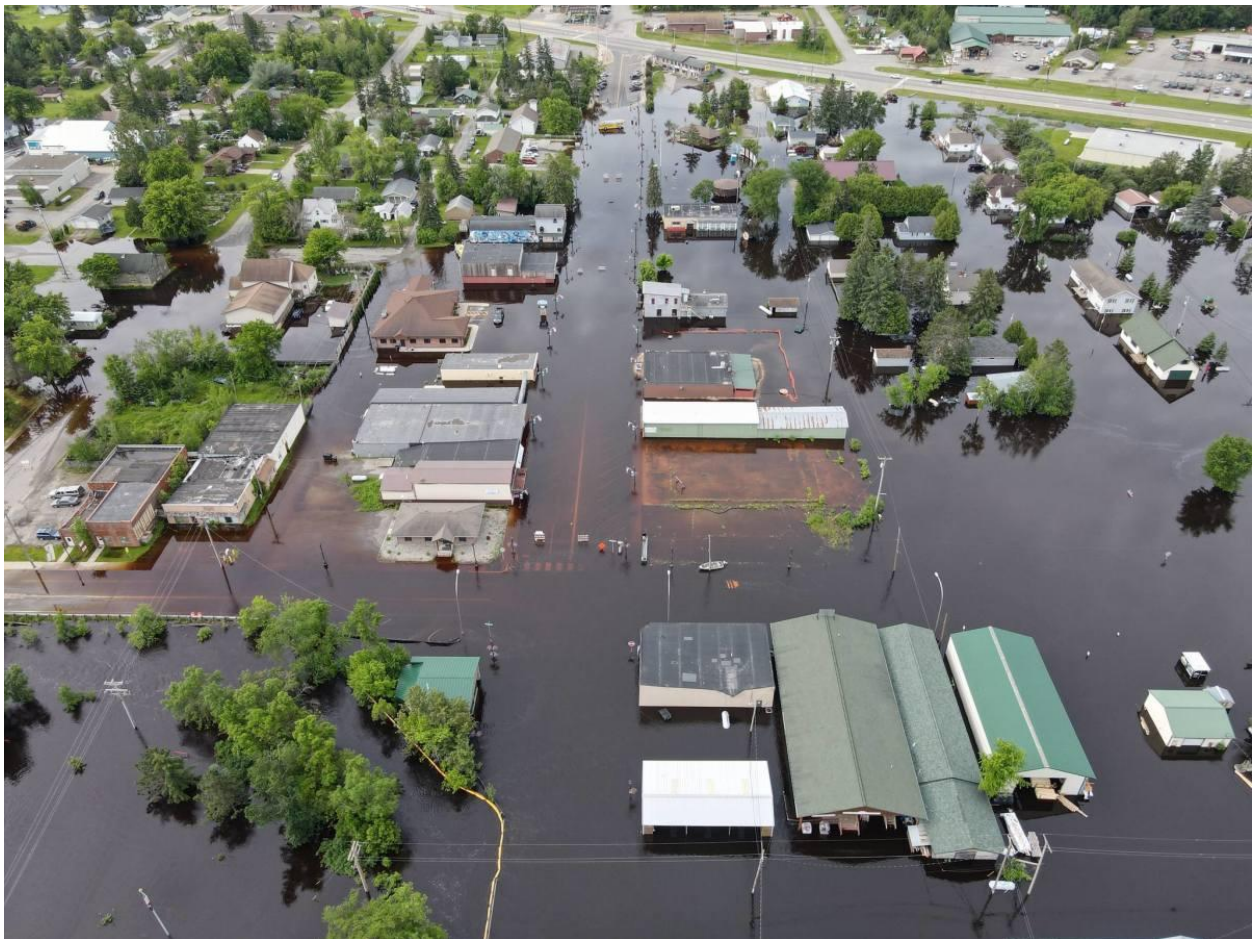
Figure 2. Flooding in Cook, MN on June 21, 2024.
